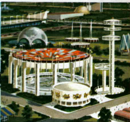
A translucent roof: New York State Pavilion.
