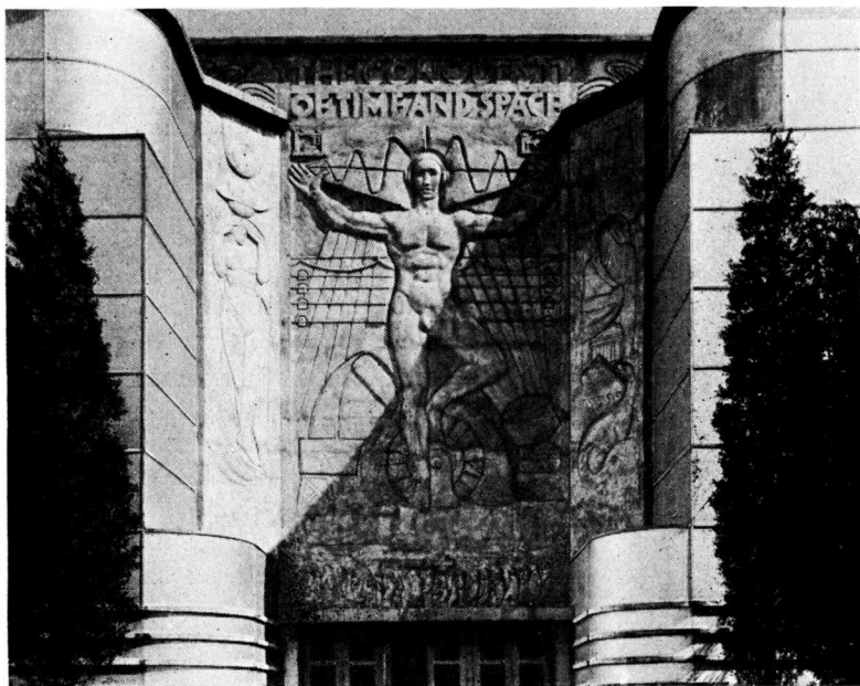
Entrance to Western Union Hall
